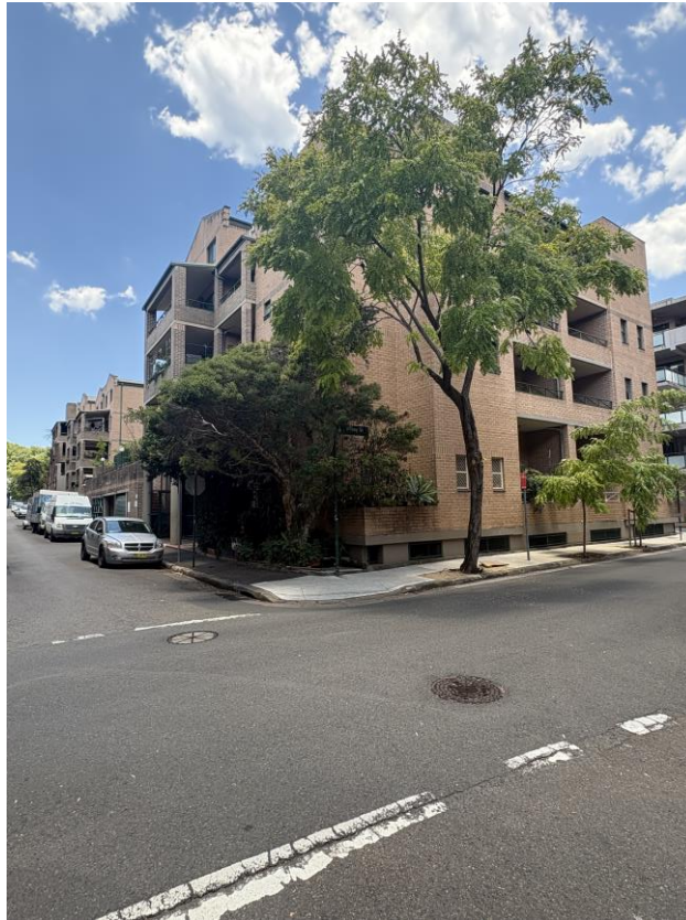
Figure 1: 39 Dangar Place, Chippendale viewed from the north-west
